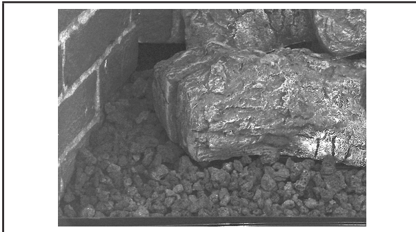
Figure 47: Installing the volcanic stone
