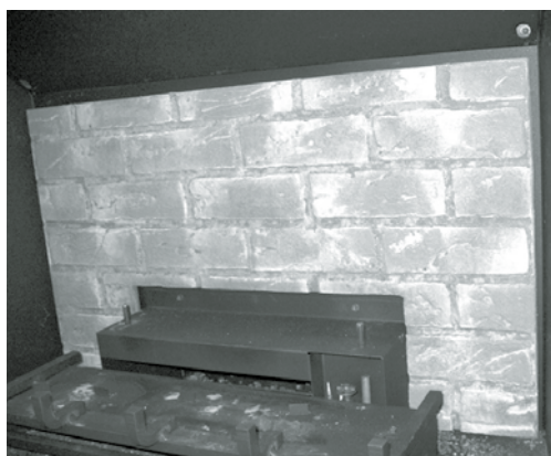
Back Panel Installed
