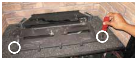
Diagram 1: Remove the left and right screws.
