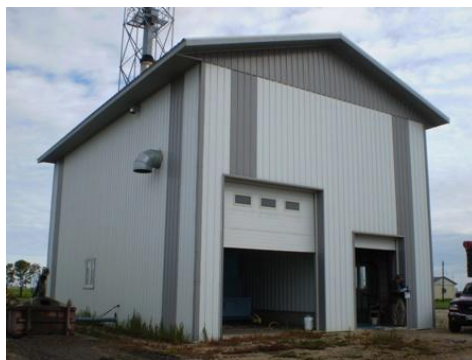
Figure 8-4: Biomass Heating System Building
