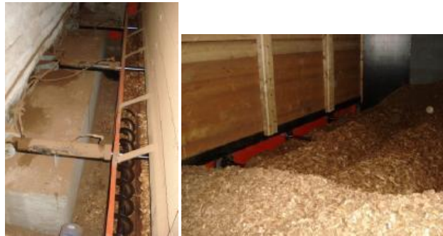
Figure 6-9: LINKA Walking floor mechanism 14
