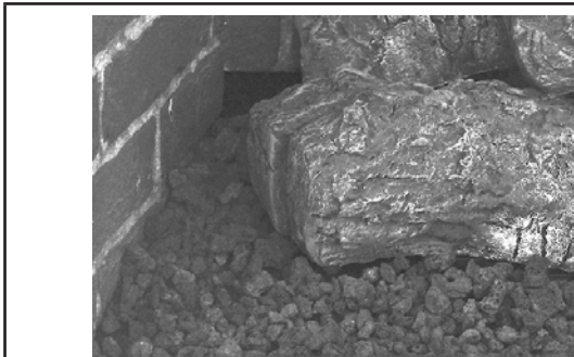
Figure 45: Installing the volcanic stone
