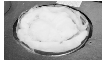
Step 3: Remove insulation from inside flue pipe.
