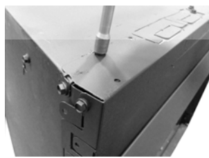
Step 1: Remove two screws from the top and side of the unit. Bend the side bracket securing tab over the edge of the unit and secure. Secure bracket to the top through the clearance screwhole.
