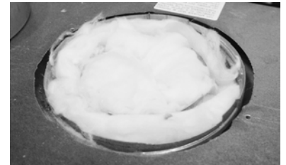
Step 3: Remove insulation from inside flue pipe.
