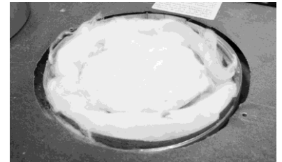
Step 3: Remove insulation from inside flue pipe.
