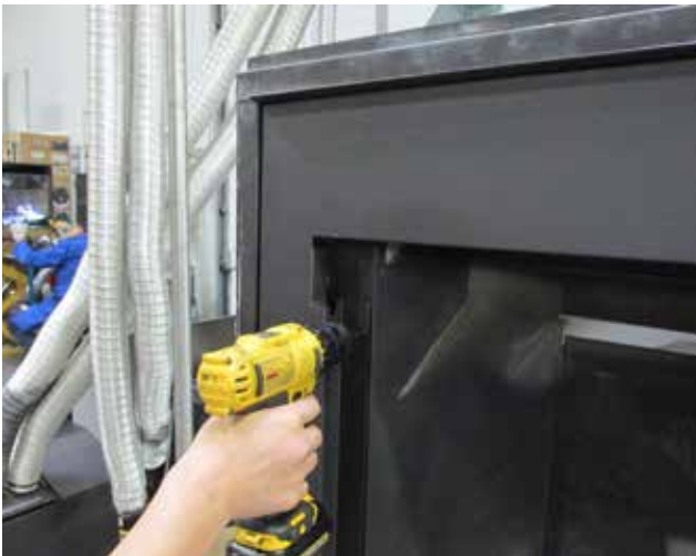
Install outer faceplate
