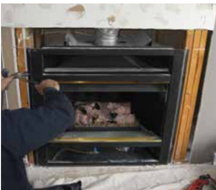
Remove unit from framing
