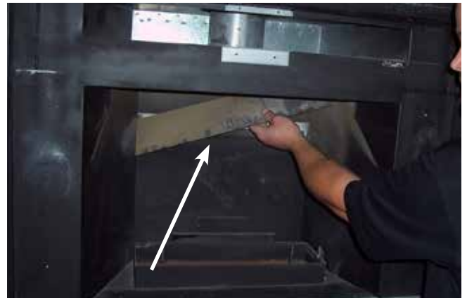
Remove rear baffle.
