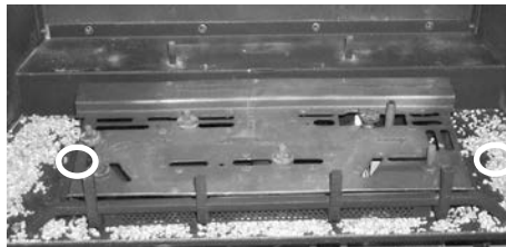
Remove 2 screws, then push burner tray to left and lift out.
