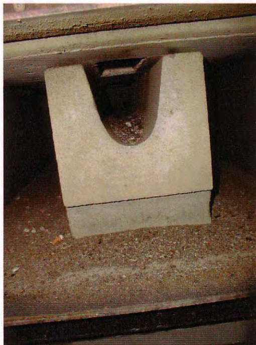
Fig. 4: - view of the boiler combustion chamber
