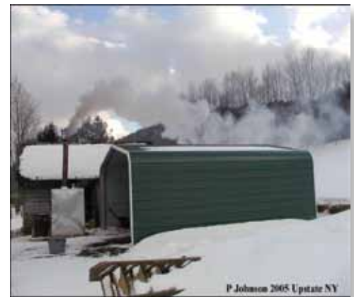
Outdoor wood boiler in Upstate New York
