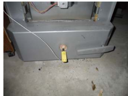
“K” type thermocouple measuring secondary chamber temperatures
