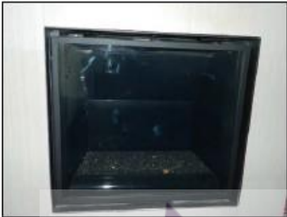
Figure 96: Glass Frame secured to the Unit
