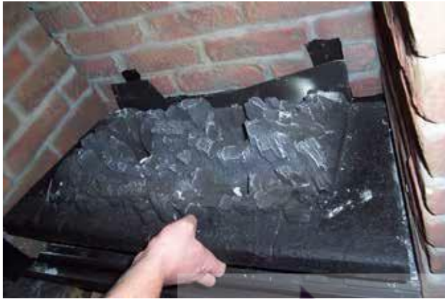
Figure 79: Burner Removal
