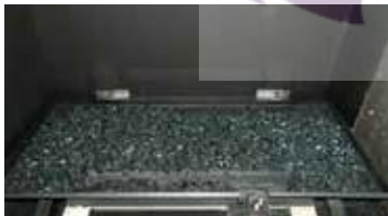
Figure 69 3) Work Crystals downwards to front edge of Firebox Floor
