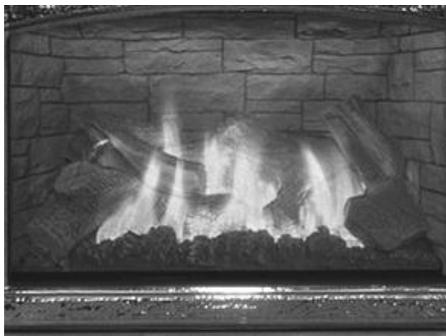
Photo 10 – Typical Burner Flame Appearance
