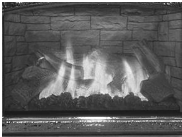
Photo 10 – Typical Burner Flame Appearance
