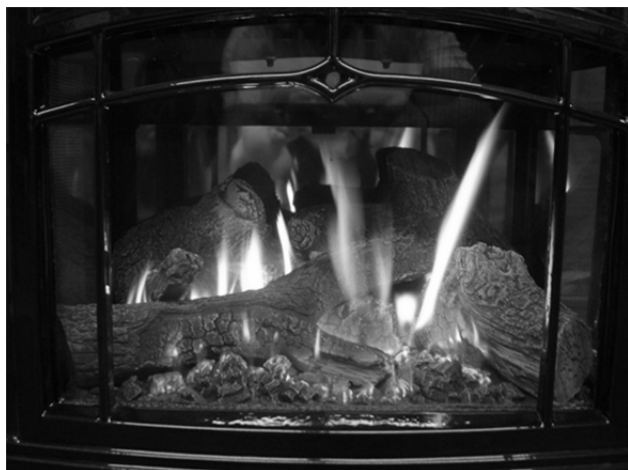
Photo 9 – Typical Burner Flame Appearance
