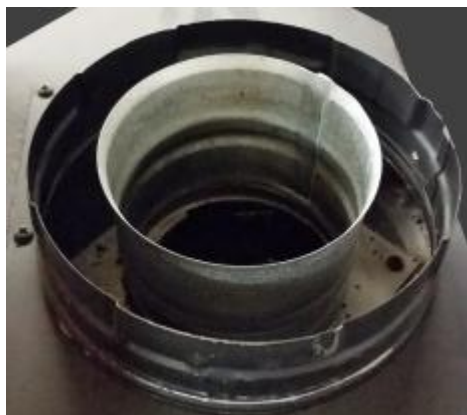
Vent Attachment Inspection – unbent and attached rings
