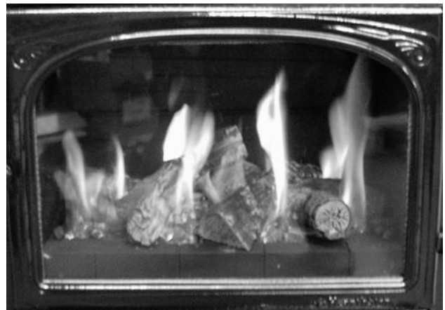
Figure 34 – Typical Burner Flame Appearance
