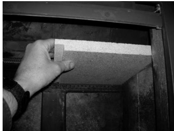
Figure 16 (cont.) - Removing/Replacing the Baffle for Inspection
