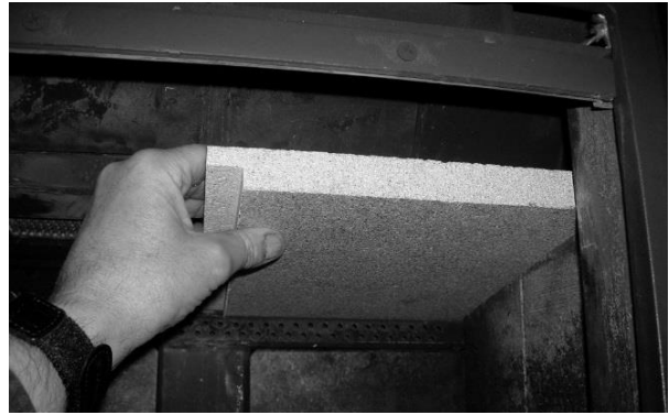
Figure 18 (cont.) - Removing/Replacing the Baffle for Inspection
