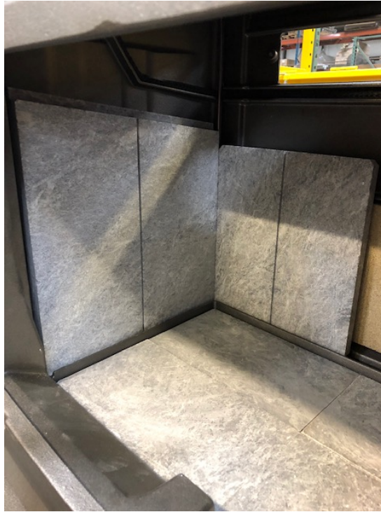
Photo 2. Left side refractory stone installed.
