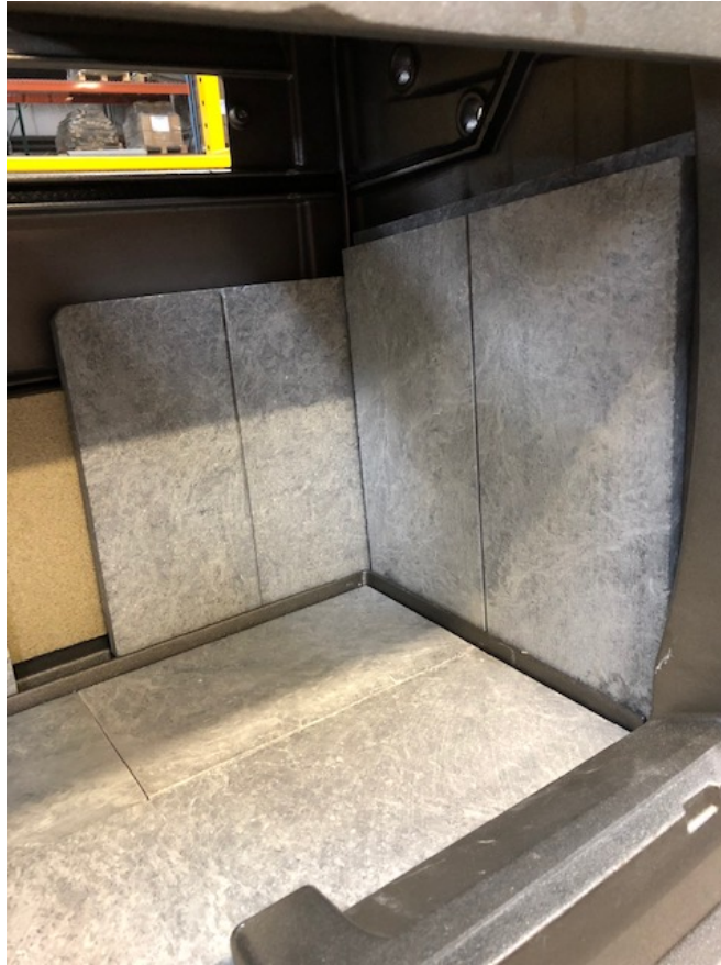
Photo 4. Right side refractory stone installed.
