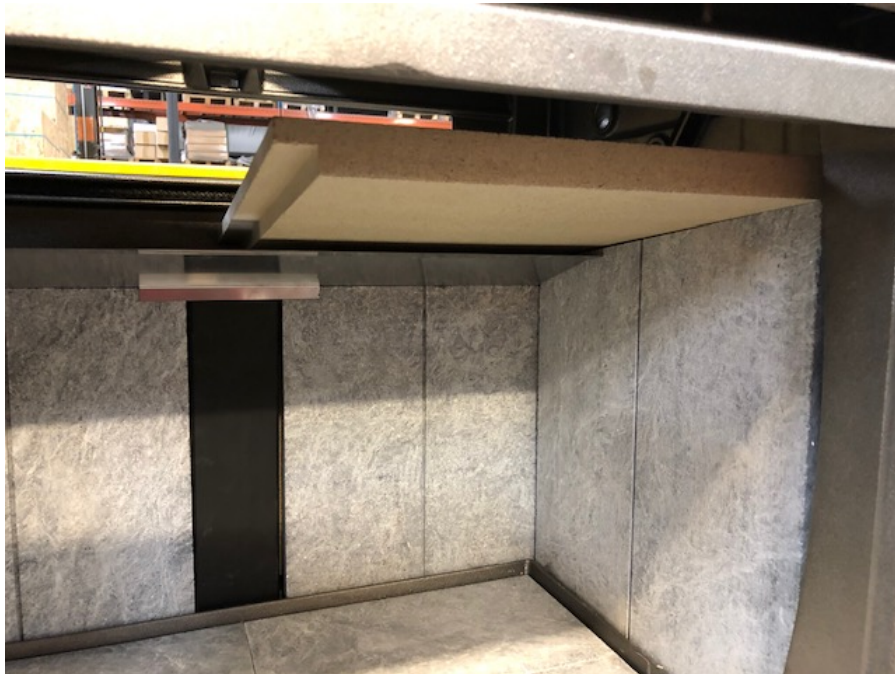
Photo 6. Right side baffle half installed.
