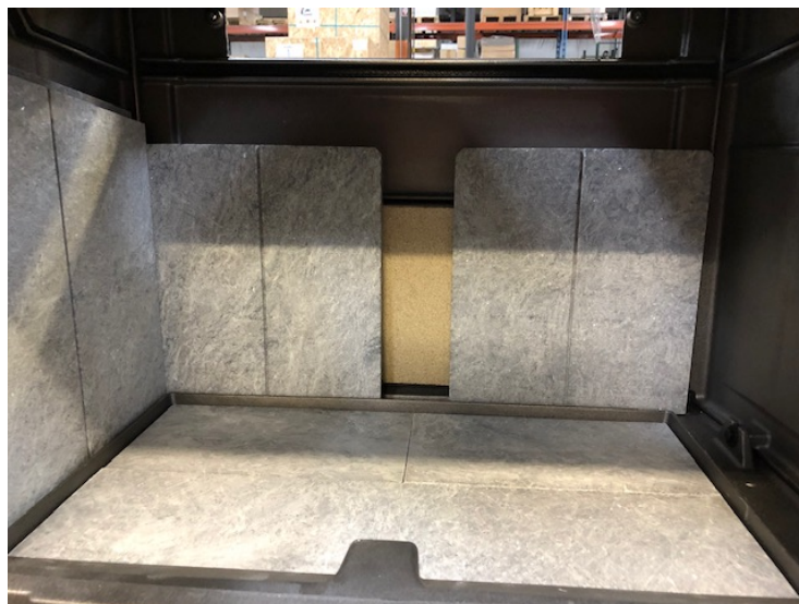
Photo 3. Right rear refractory stone installed.
