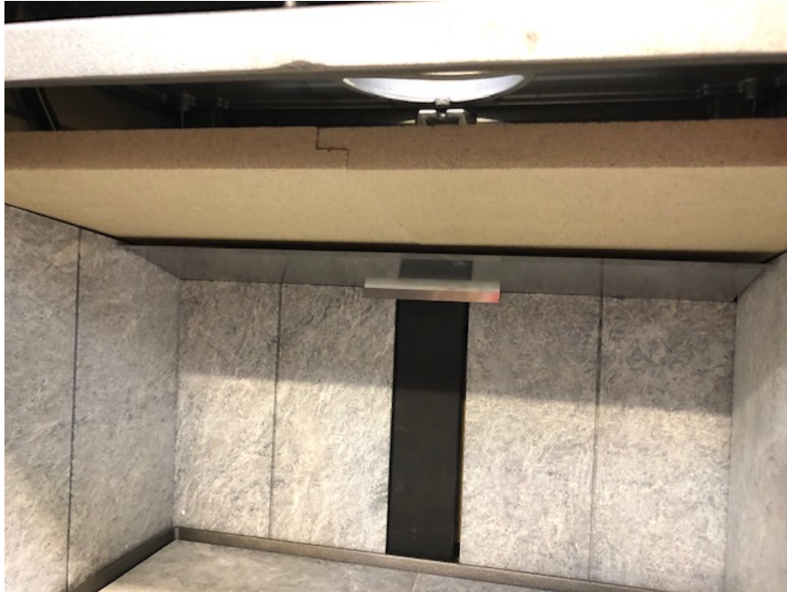
Photo 7. Vermiculite baffles installed.
