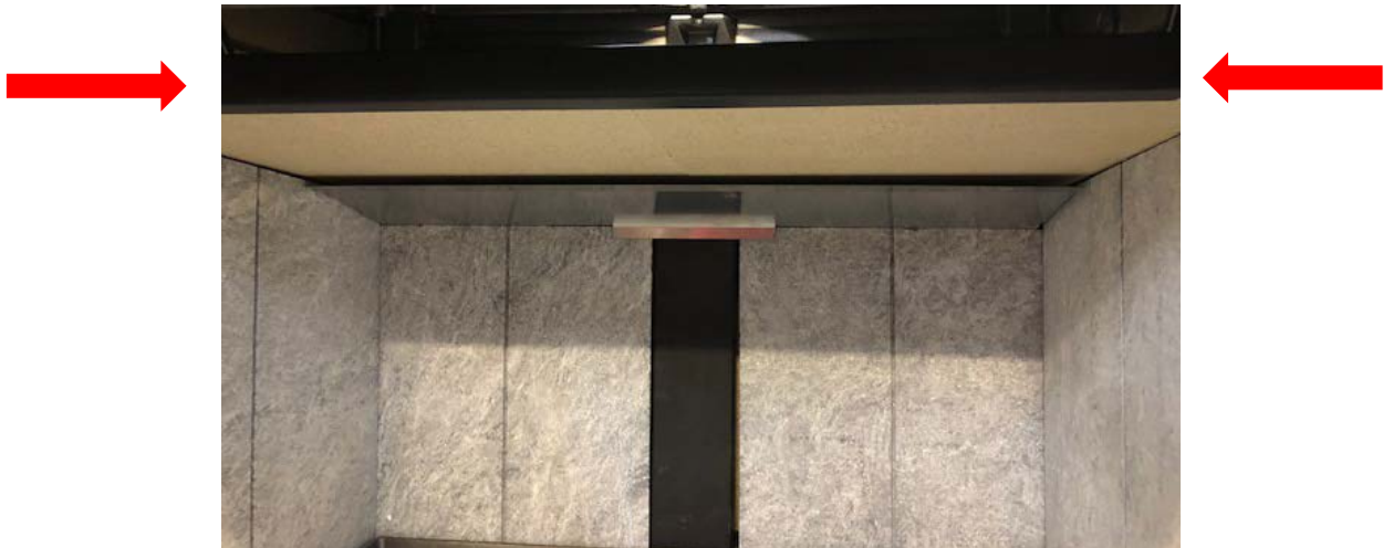
Photo 8. Baffle guard installed.
