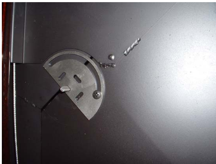
Photo 13: Restrictor Fully Closed
