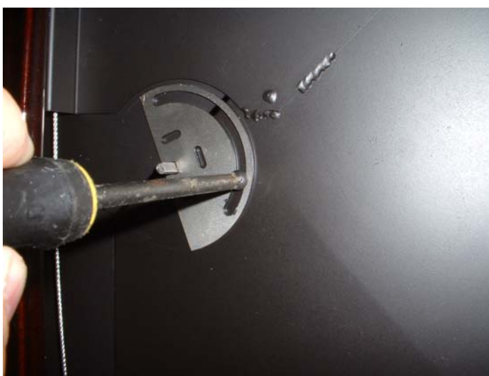
Photo 14: Restrictor Fully Opened (no restriction)
