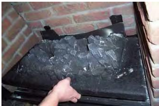
Figure 79: Burner Removal
