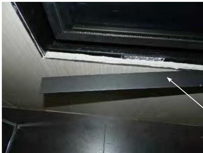
Figure 101: Top View - Sliding trim into place
