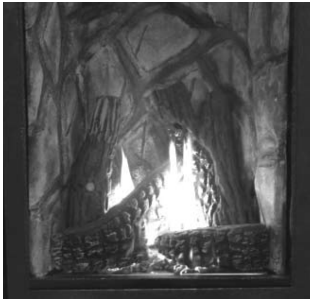
Figure 53 - Burner Flame Appearance
