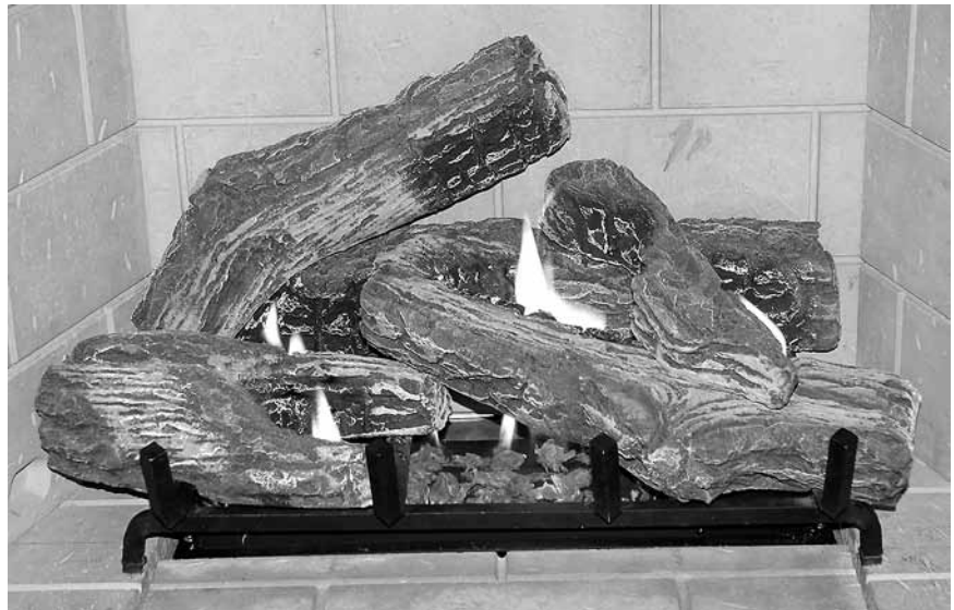
Figure 14 - Burner Flame Appearance
