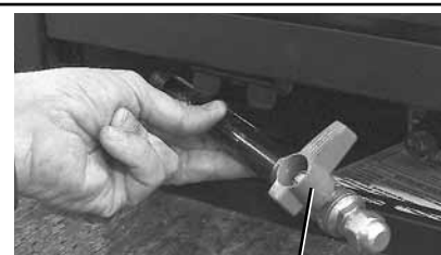
Length of pipe with attached Gas Shut-Off Valve in OFF position (gas line CLOSED)
