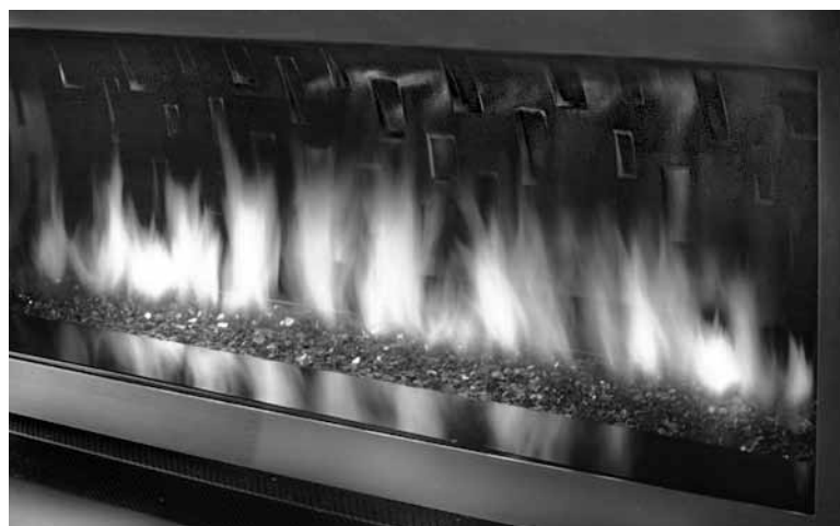
Figure 53: Proper Flame Appearance
