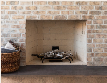
Existing Fireplace Before
