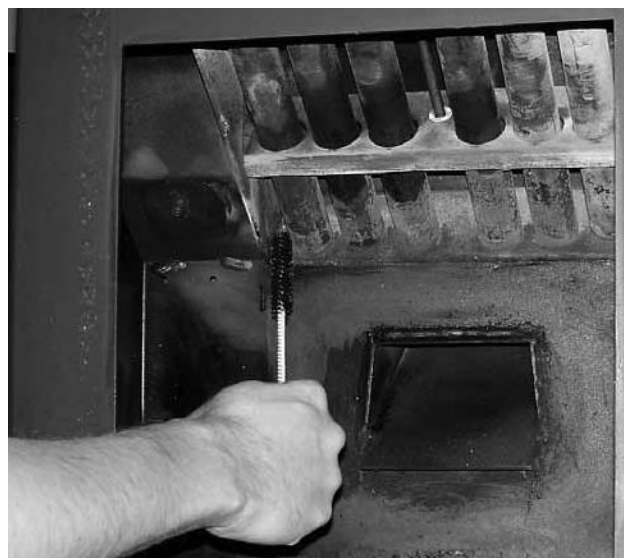
Figure 25 - Clean Behind Tube Scraper
