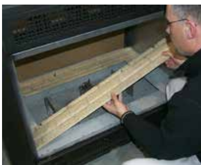
Remove the 2 Long Base Brick Panels
