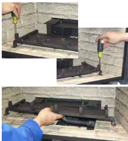
Diagram 1: Remove the left and right screws and then slide the burner/grate assembly to the left and lift out.
