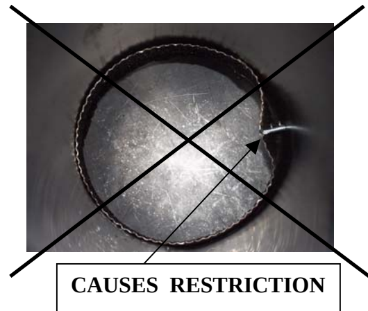
FAULTY INSTALLATION
