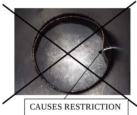
IMPROPER INSTALLATION
