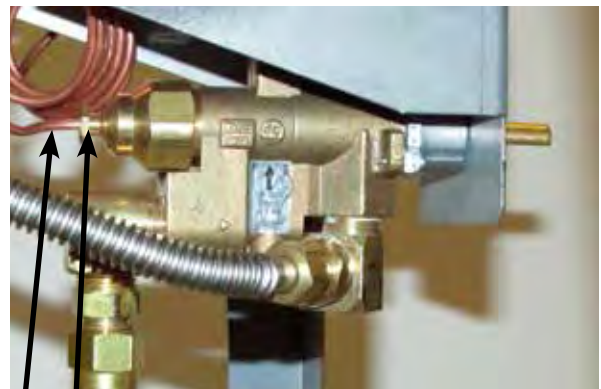
Thermocouple Loosen nut
