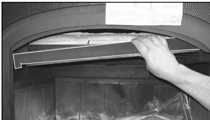
Figure 4.5 Removing Baffle Protection Channel
