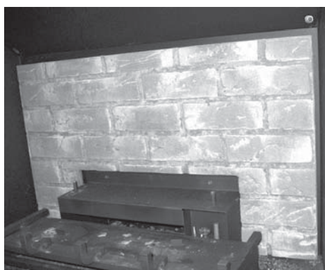
Back Panel Installed
