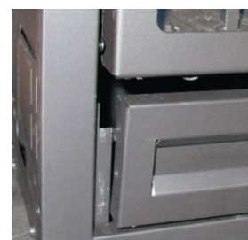
Installation of lower Louver/Flush Panel
