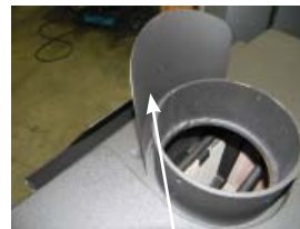
Installed Pipe Shield
