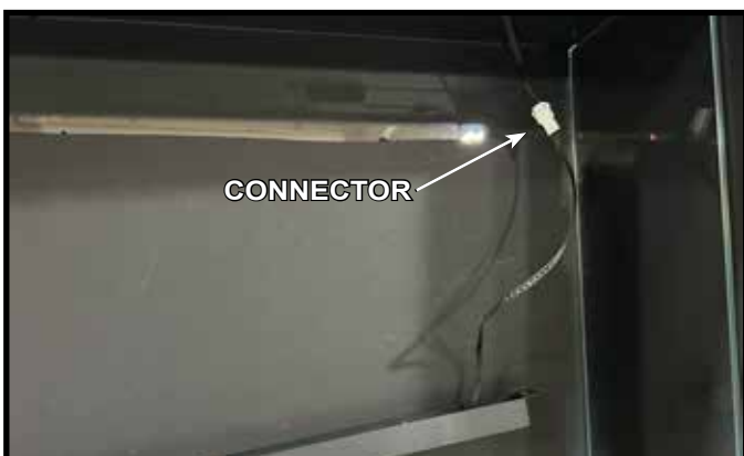
Figure 4 Downlight Connector
