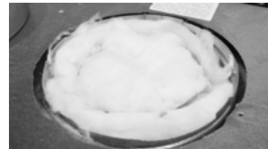
Step 3: Remove insulation from inside flue pipe.
