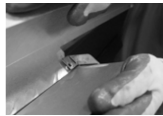
Step 1: Carefully bend up the two (2) tabs on the heat shield at a 90° angle from each opposite joint and then the foot of the Standoff at approximately a 45° angle.
