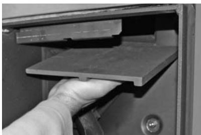
Fig. 118 Cleaning the baffle plate
