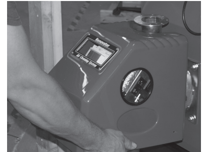
3. Lift the cover off the burner.
