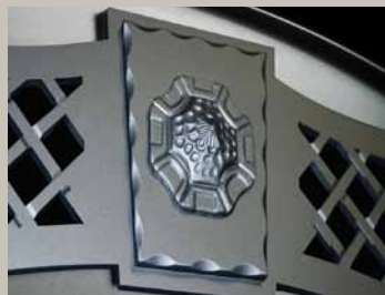
Wrought iron keystone and lattice design
